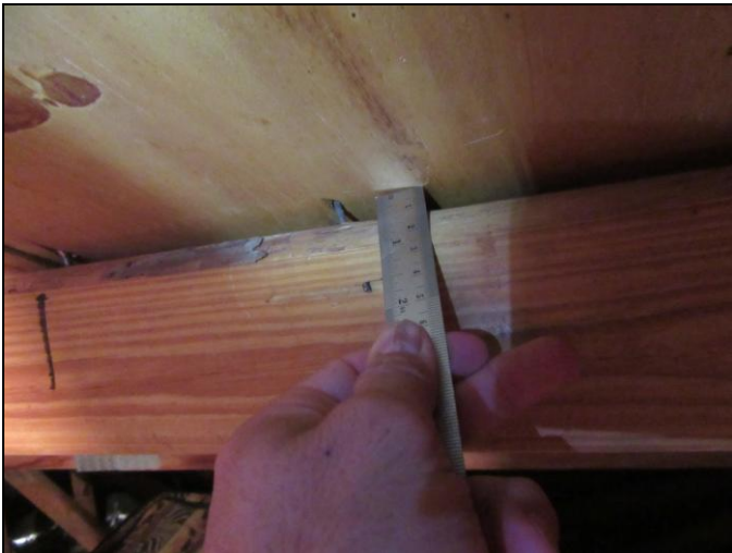
Roof Deck Fastener 6d nails
