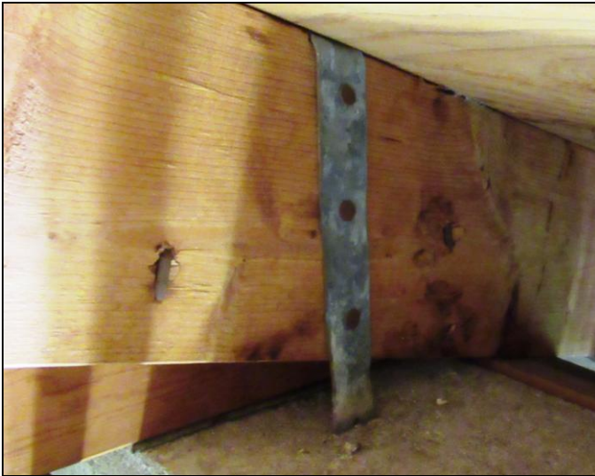
Roof To Wall Connection – Clips Min. 3 nails in metal connector
