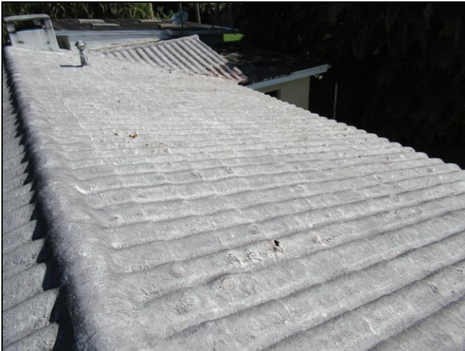
Roof Covering Picture
