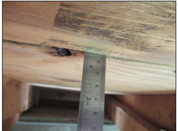
Roof Deck Thickness 1/2" Decking
