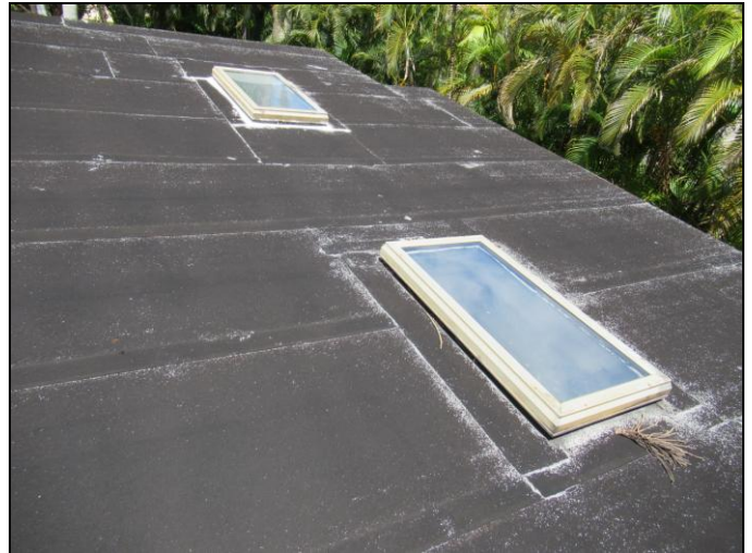
Roof Covering Picture
