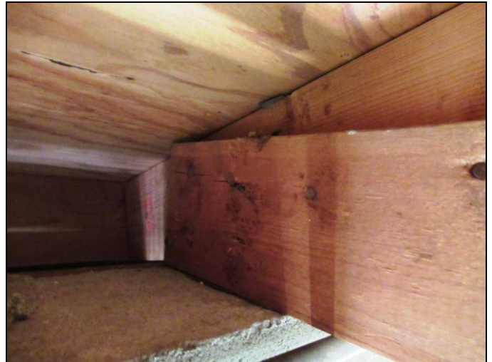
Roof To Wall Connection – Clips Min. 3 nails in metal connector
